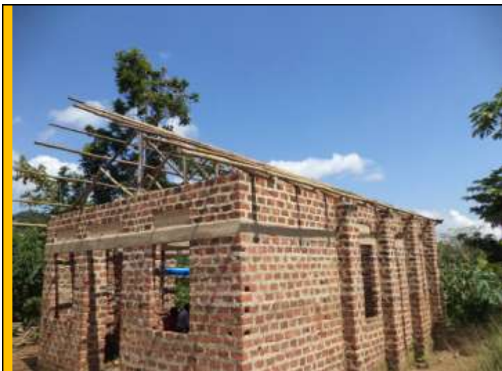
Fixing Timber on church for roofing
