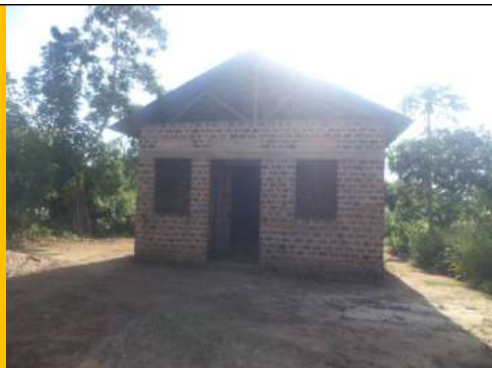
After roofing the church with iron sheets.
