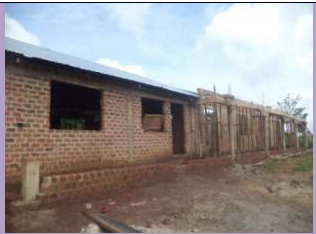
Our School structure under Construction
