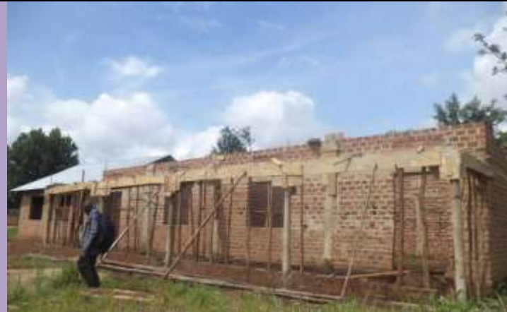
On going work for school construction
